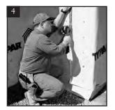
the inside and outside corners. Tape all vertical and horizontal seams, and penetrations.
